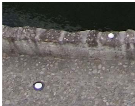
Figure 3: Marked control point and laser scan target from oblique aerial view
