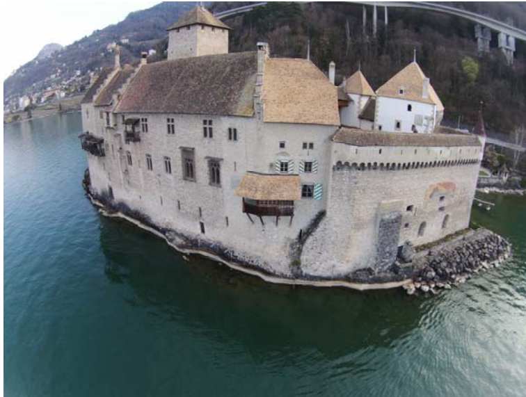
Figure 18: Example of one DJI Phantom2 Vision image from the lake side, captured by boat operation
