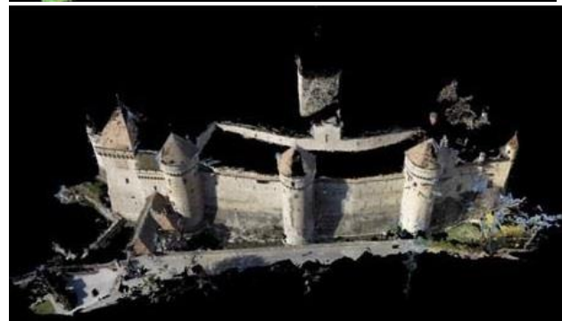
Figure 21. Results of the bundle adjustment. Automatic tie points, GCPs, and camera centres shown in rayCloud Editor (top) and the resulting dense point cloud (bottom)
