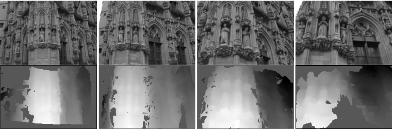
Figure 3. Top: Four images used in the wide-baseline experiment. Bottom: depth maps for these images (dark pixels indicate low consistency regions).
