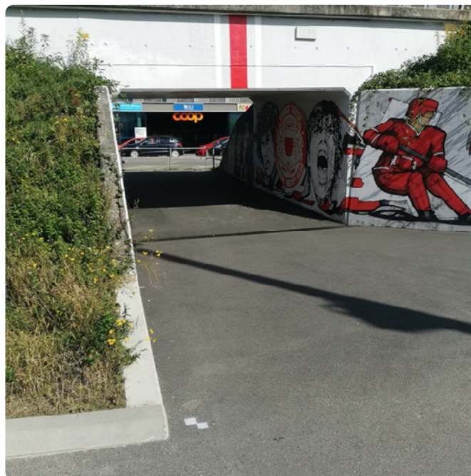
Figure 16: The tunnel on the Vaudoise area.
